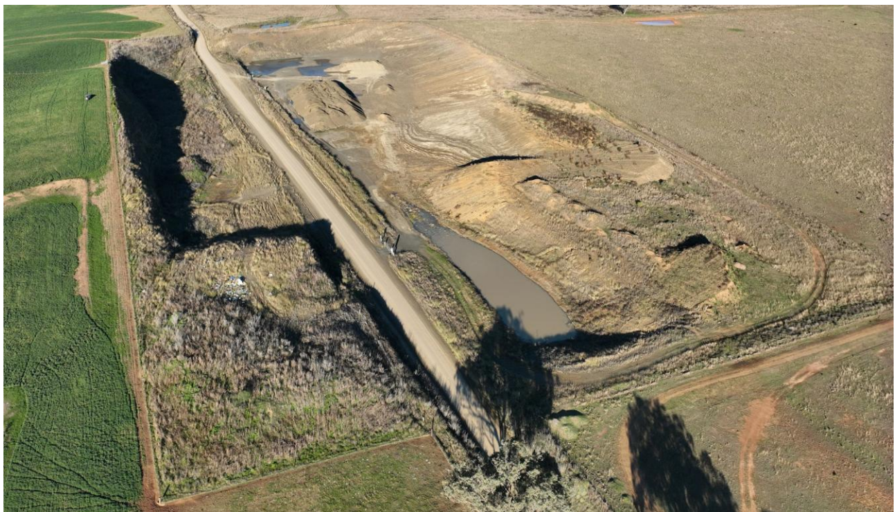
Plate 2.3 – Oblique aerial drone image of TfNSW quarry (left) & TRC quarry (right) separated by Spains Lane (centre), June 2024.
